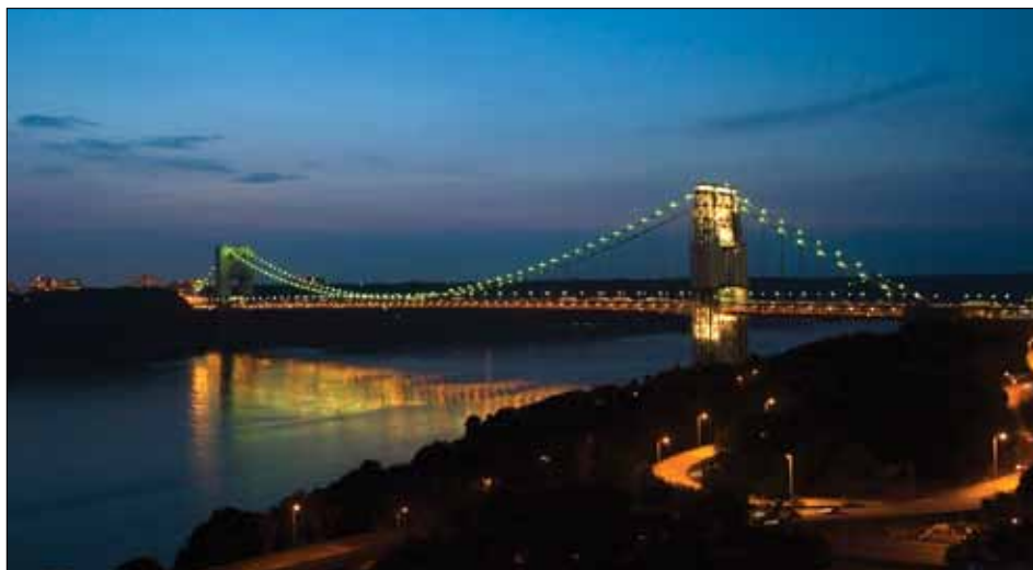
Our bridge at dusk
